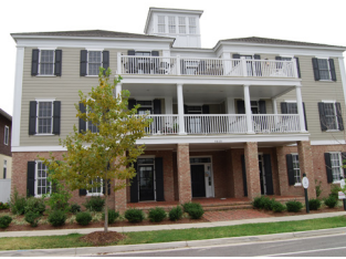
Figure 1.5 Example of an Upper MMH type, 3-story large multiplex within a residential neighborhood.
