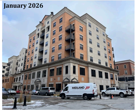
Currently under construction
